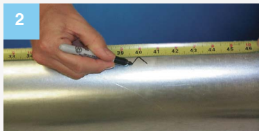
On raw end of provided Pipe, mark the distance to be spanned less 1" .
