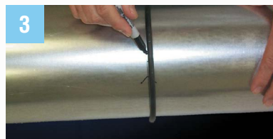
3 Use provided O-ring to mark for cut.
