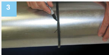
Use provided O-ring to mark for cut.
