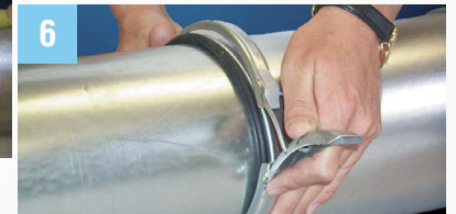
6 Snap QF Clamp over O-ring and one end of Quick-Fit Sleeve.
