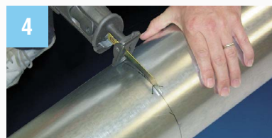
4 Drill access hole, then cut Pipe with saw.
