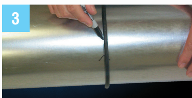
Use provided O-ring to mark for cut.
