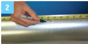
On a Pipe, mark distance to be spanned less 4".
