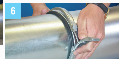
Snap QF Clamp over O-ring and one end of Quick-Fit Sleeve.
