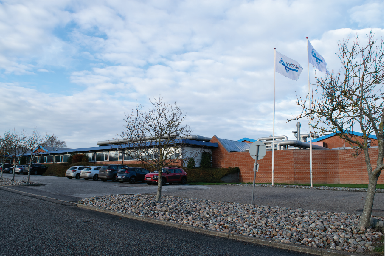
Nordfab Europe sales and manufacturing facility in Assens Mariager. Denmark.
