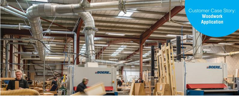
When Tom Howley, manufacturer of luxury kitchens, had to replace older machinery with newer, they contacted Nordfab's distributor, Extractly Ltd for help. Extractly Ltd used Nordfab ducting for this project where they had to reconfigure the ductwork arrangement and integrate Ecogate equipment. The results were impressive; reduced noise impact and a much improved energy-efficient ducting system.
