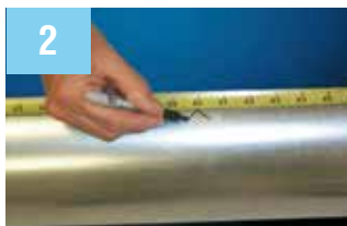
2 Mark distance to be spanned less 100 mm.
