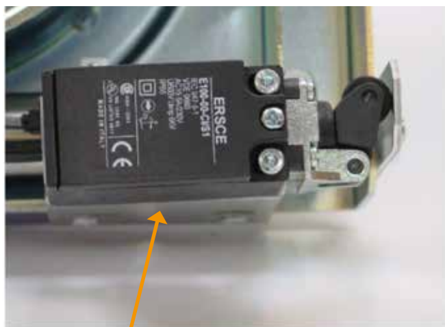
Micro breaker attached on damper.
