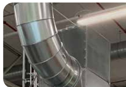
QFS Segmented Bends allow airflow direction change in a run of duct.
