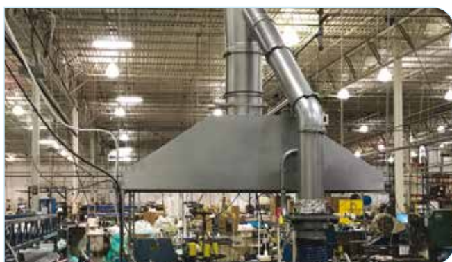
Example of a Transition from rectangular to round
