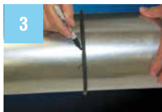
3 Use O-ring provided and mark for cut.
