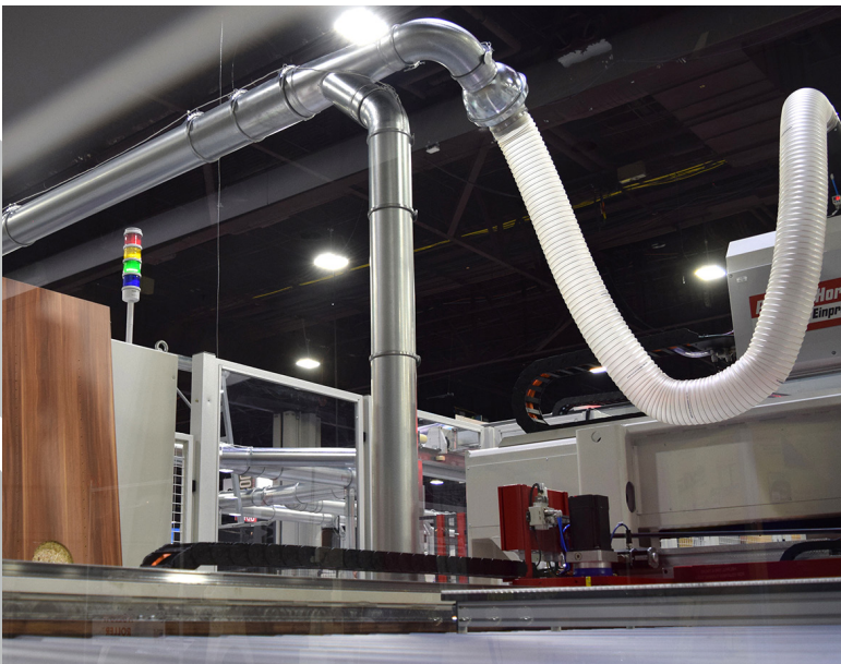
Above: A QF Ball Joint is shown in a QF duct line installed on woodworking machinery. Nordfab provides a full range of PU Hoses.
