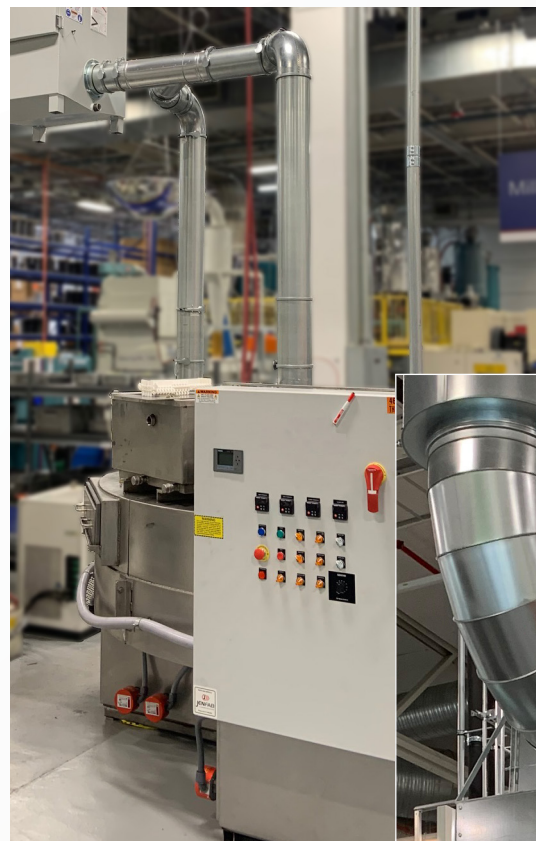
QFS Ducting installed on machines in automotive parts manufacturing facilities
