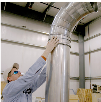
Lift pieces into place
