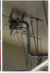
The most effective method of limiting the exposure to diesel exhaust is the Exhaust Source Capture System. Inside the fire station a pneumatic nozzle, connected via hose to a ducting system above, is attached to the Fire truck's tailpipe where it captures the fumes and then easily pulls them out of the building.
