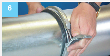
Place QF Clamp over the O-ring and end of Quick-Fit Sleeve.
