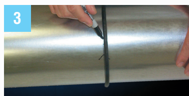
3 Use O-ring provided and mark for cut.
