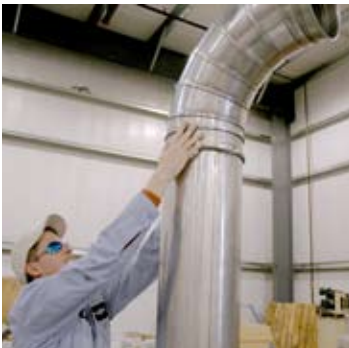
Lift pieces into place
