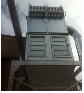
Important note: Fires and dust explosions can be caused by various ignition sources including sparks and optimum dust concentrations etc. We recommend fitting dust collectors with explosion vents and locating them outside of buildings to reduce the risk of damage to property and personnel in the event of an explosion or fire.
