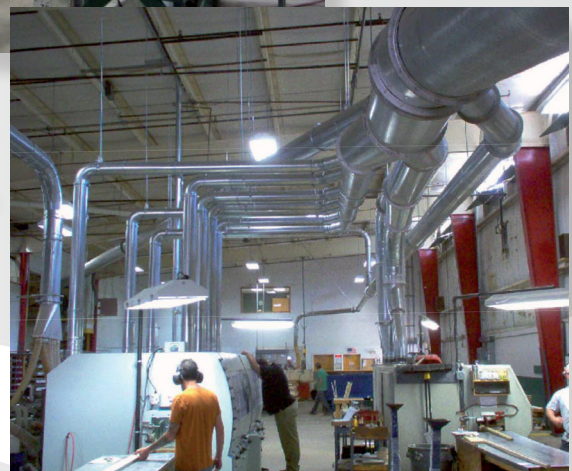
Right: After installation of Nordfab ducting.
